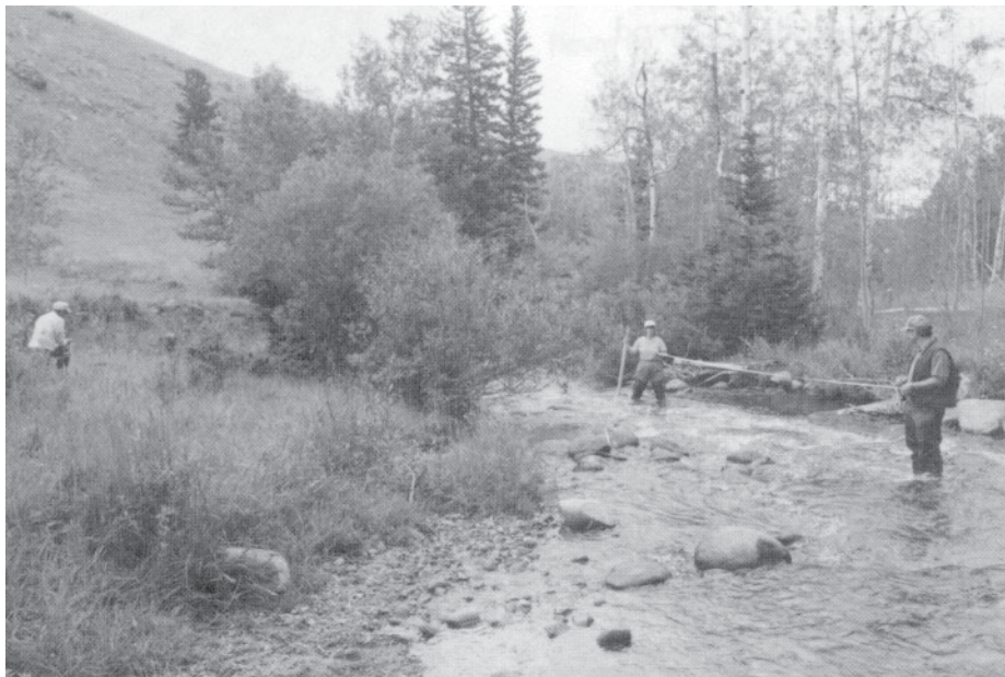
Figure 50. Measuring along the channel centerline and staking.
