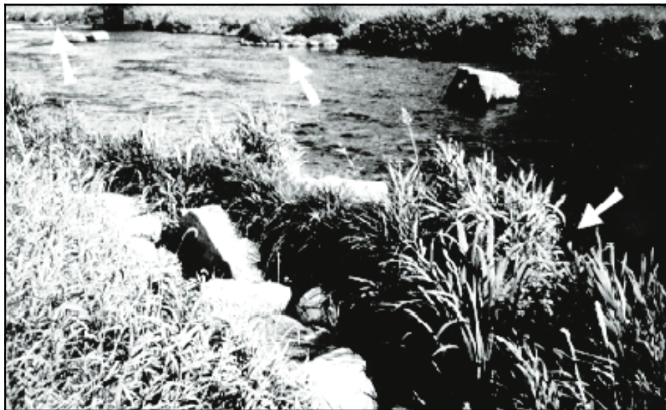
Figure 22. Photo of coir geotextile roll and rocks with wetland plants serving as a deflection system and providing aquatic habitat on a German stream (Note that two can be seen on opposite bank also) (Photo courtesy of Bestmann Ingenieurbiologie, Wedel, Germany)
