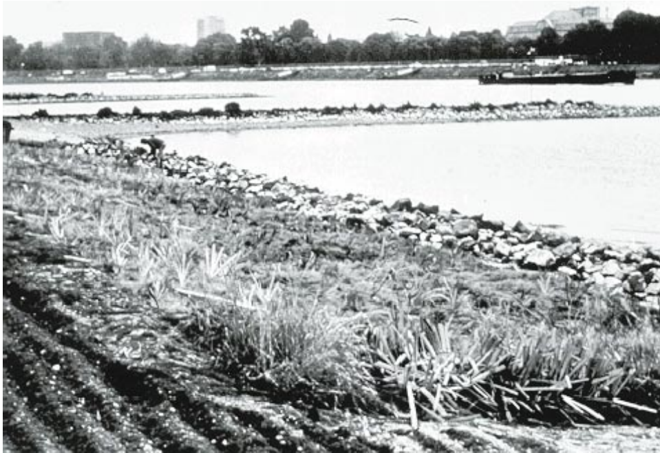
Figure 12. System of bioengineering treatments such as geotextile coir mats with planted vegetation on them placed above a rock roll toe and between large rock transverse dikes
