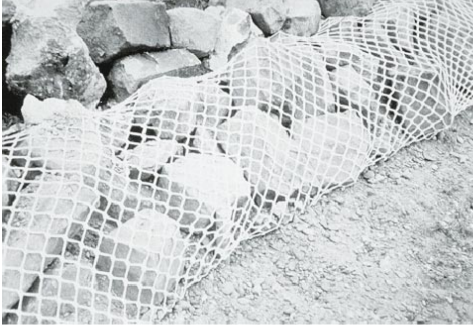
Figure 11. Rock roll used as toe protection on a bioengineering project, Rhine River, Germany, in city of Dusseldorf
