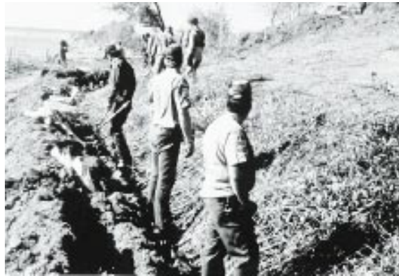
b. Placing woven wire over willow brush
