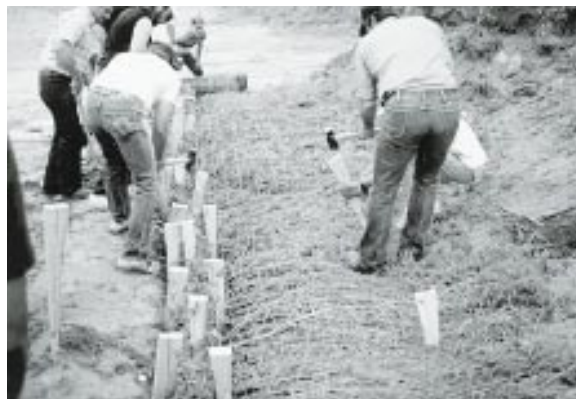
c. Stretching woven wire tight and securing by wedge-shaped stakes (Also, wattling bundles are then laid over the top of basal ends of willow in trench and secured tightly with wedge-shaped stakes)
