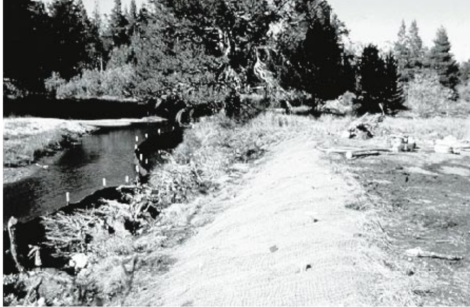
Figure 38. Burlap and coir woven fabric laid over sedge and grass seed, Upper Truckee River, California (Note that fabrics were keyed in at top and bottom in trenches and securely staked with wedge-shaped stakes) (Photo courtesy of Interfluve, Inc.)
