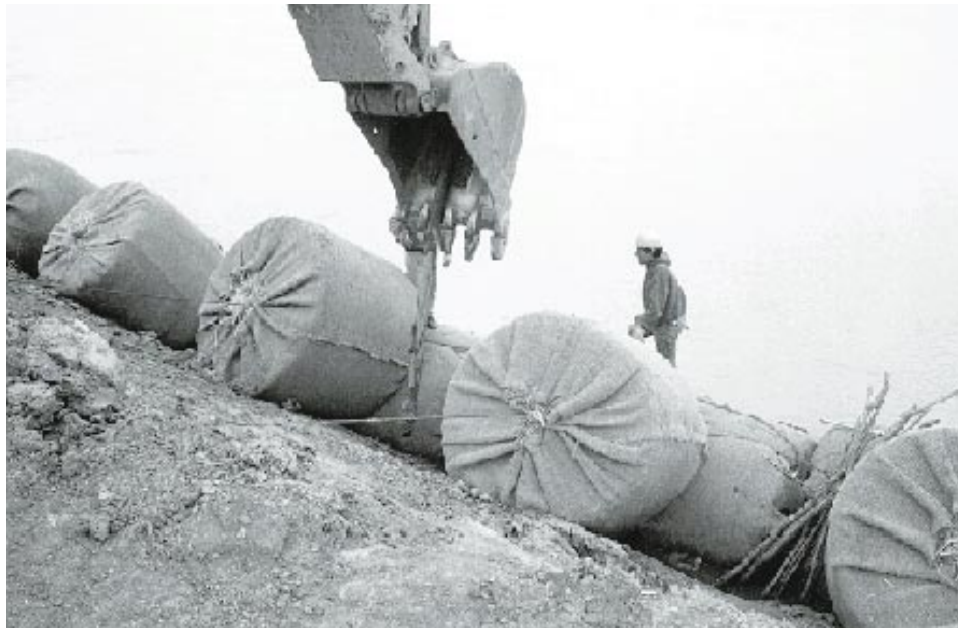
Figure 36. Use of “The Stinger” to create pilot holes for dormant willow posts on upper Missouri River (CE project, Omaha District)
