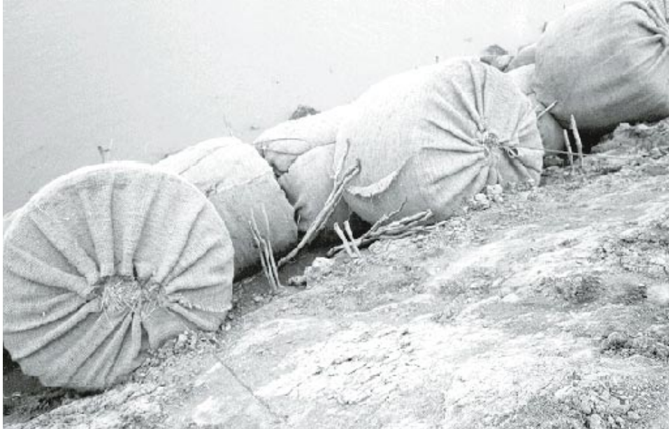
Figure 10. Vegetation in the form of dormant willow posts (discussed later) placed landward of rock and hay bale toe
