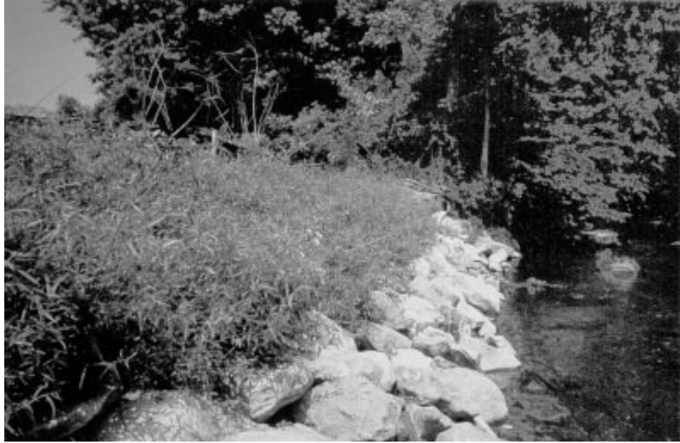
Figure 30. Brush layering with willow and dogwood branches after one growing season; installed above a rock toe (to prevent undercutting) on the Little Patuxent River, Maryland (from Bowers 1992)
