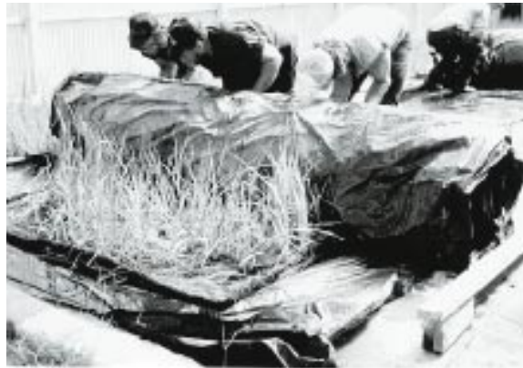
b. Emergent aquatic plants established on a coir fiber mat being rolled up in WES nursery ready for transport to bioengineering site
