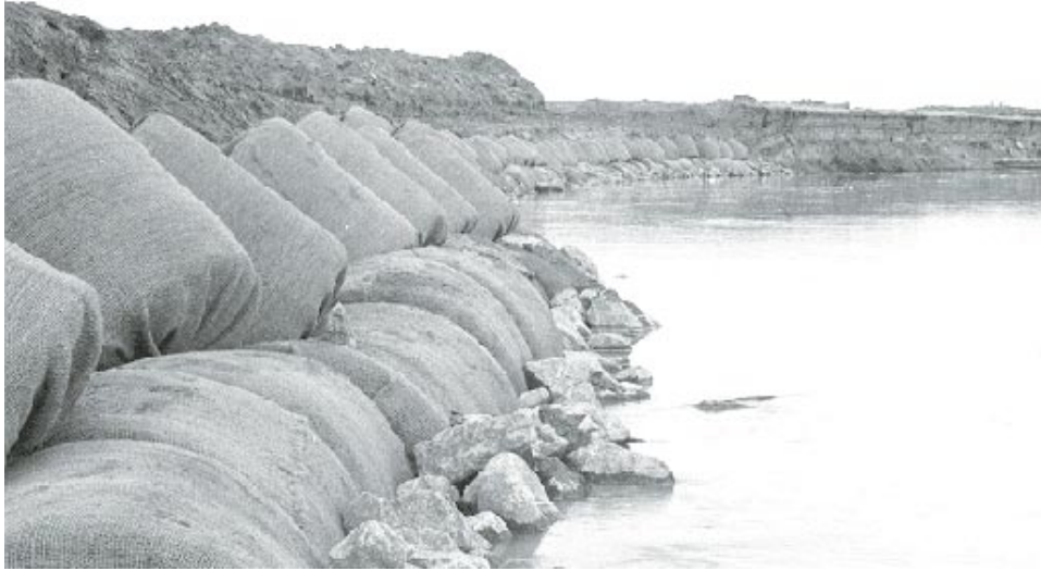
Figure 9. Photo of bioengineering project on upper Missouri River where large rock (1.5 tons/lin ft) was used as toe protection below large coir-covered hay bales, also forming part of toe
